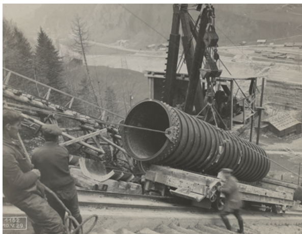
Construction of the pressure pipeline in Partenen, 1929, Photograph: illwerke vkw
